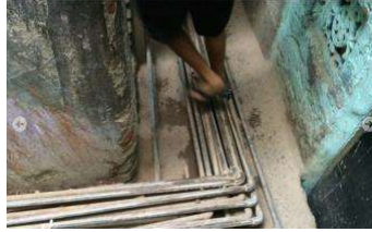
In the northern half of IKV, households access water through a network of privately installed, illegal pipelines that tap the formal water supply
